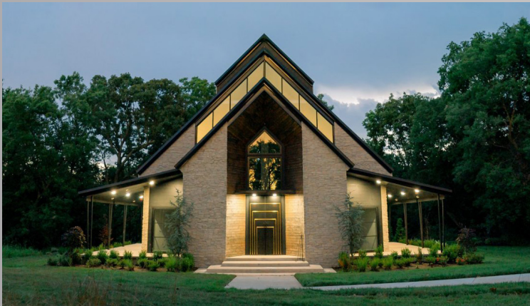
PROJECT: OSAGE HOUSE FIRM: JOHN STARNES, ARCHITECT CONTRACTOR: N/A LOCATION: CAVE SPRINGS, AR
