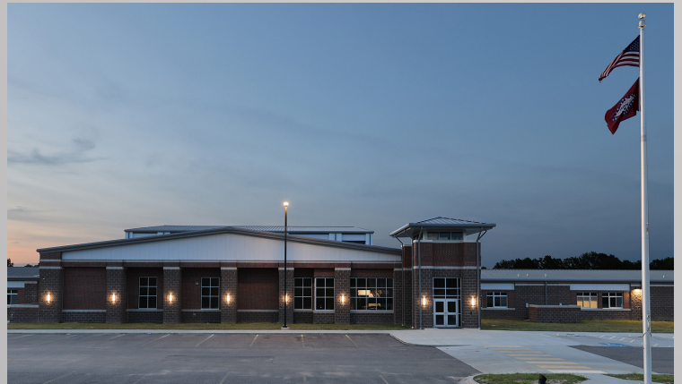
PROJECT: POCAHONTAS ELEMENTARY SCHOOL FIRM: BRACKETT-KRENNERICH ARCHITECTS CONTRACTOR: NABHOLZ CONSTRUCTION LOCATION: POCAHONTAS, AR
