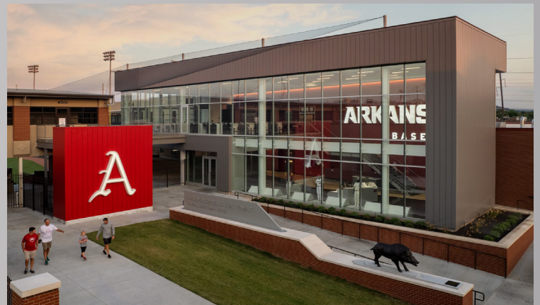
PROJECT: J.B. AND JOHNELLE HUNT RAZORBACK BASEBALL DEVELOPMENT CENTER FIRM: WER ARCHITECTS CONTRACTOR: KINCO CONSTRUCTORS LOCATION: FAYETTEVILLE,, AR
