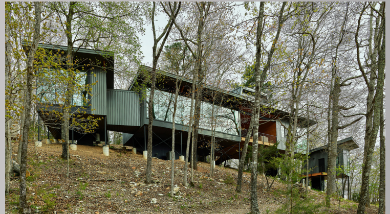
PROJECT: GRIST MILL CABIN FIRM: MODUS STUDIO CONTRACTOR: MASWORKS CONSULTING LOCATION: ROGERS, AR
