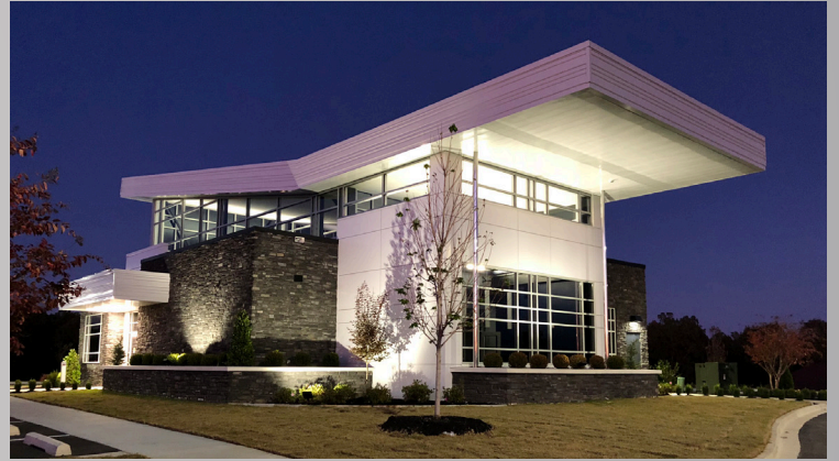
PROJECT: SUCCESS CREDIT UNION FIRM: BRACKETT-KRENNERICH ARCHITECTS CONTRACTOR: BAILEY CONTRACTORS, INC. LOCATION: PARAGOULD, AR
